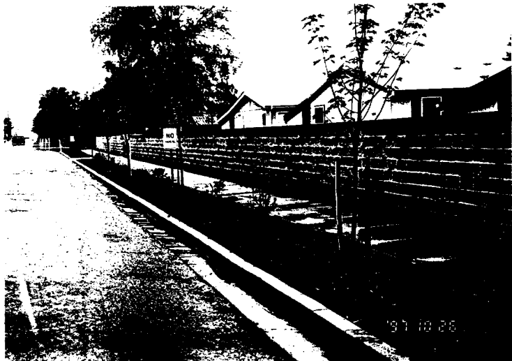
Exterior 5' block wall required by Newberg City planners
