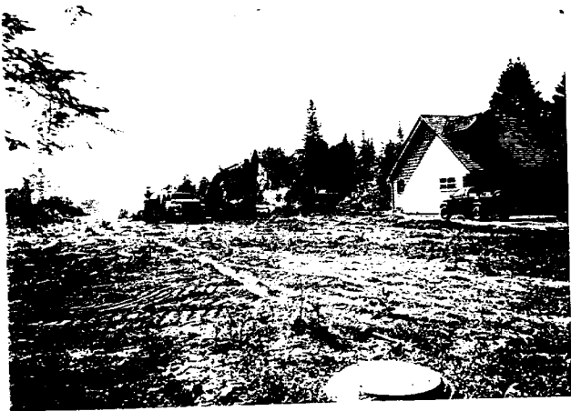
South Side of Woods Home - After Clear Cutting ON Phase II
