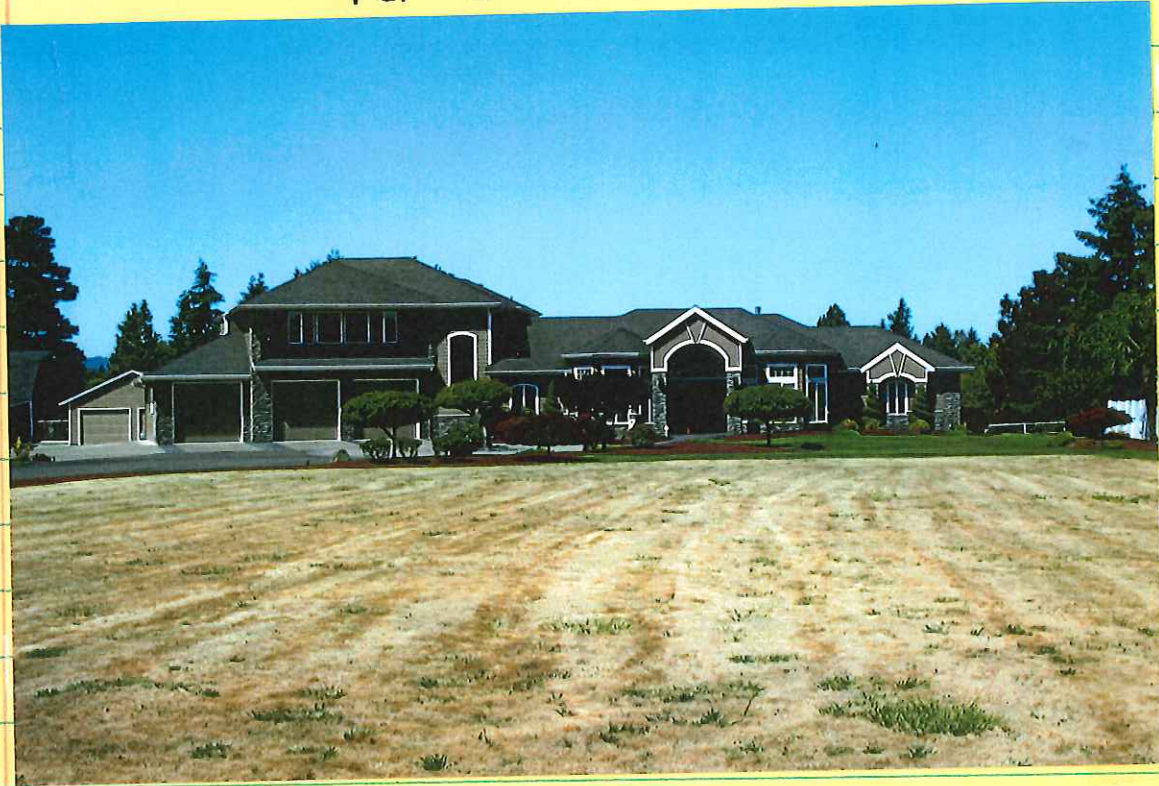
Front view from Verda of home at 4875 Verda. Fourth house south of Dearborn on west side of Verda on ridge line.
