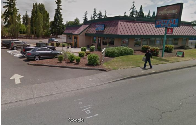
Below: Overly wide curb radii
