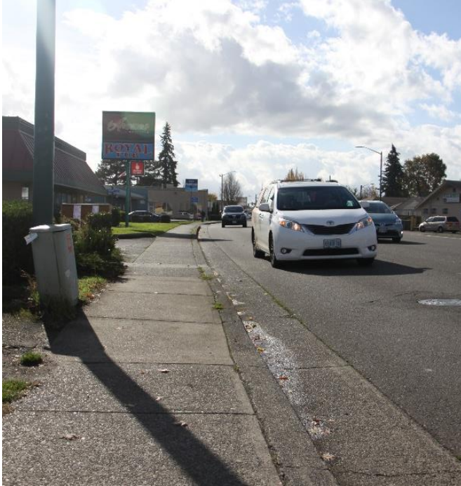
Figure 10 – “Needs Improvement” Sidewalk
