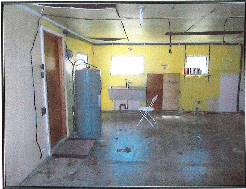
Attached garage. (A15-121)
