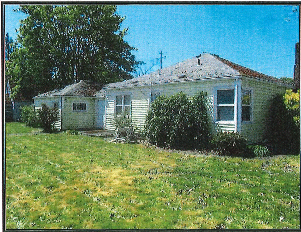
Rear view of subject's dwelling. (A15-131)
