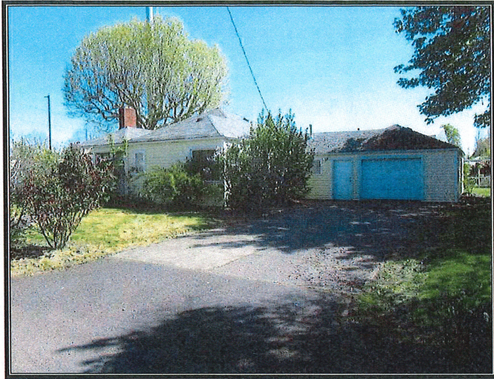
View of dwelling, attached garage, and south driveway. (A15-120)
